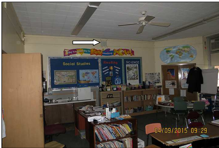
Room 210 – Classroom (arrow points to antenna)
